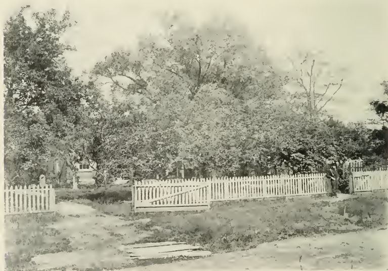
Terminus of Mohawk & Hudson Railway, Crane Street, Mt. Pleasant.
